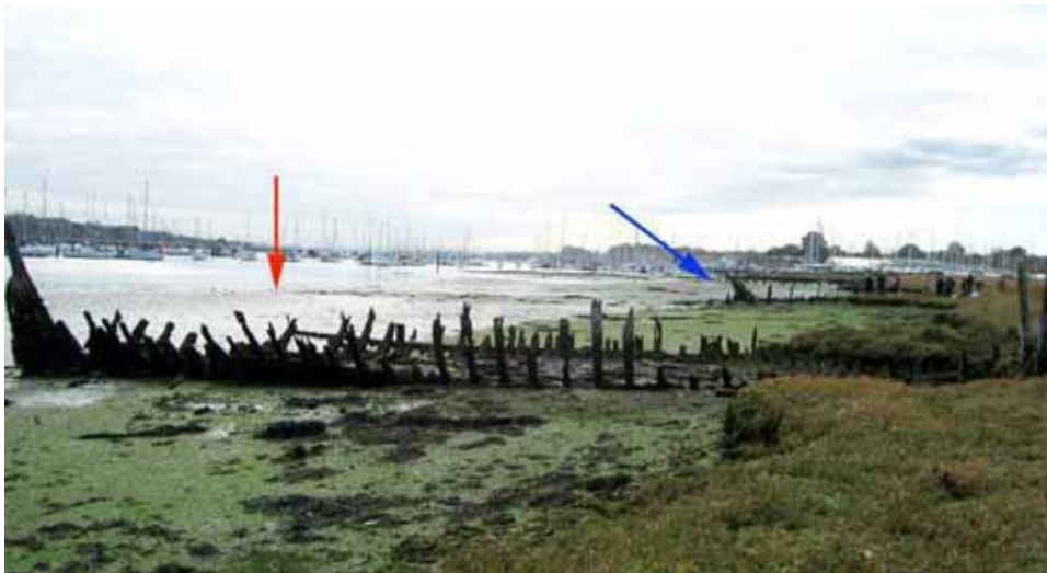
Figure HAM051- 2 The remains of HAM051 (red arrow) with HAM037 in the background (blue arrow). The embankment can be seen on the right of the photograph (looking south)
