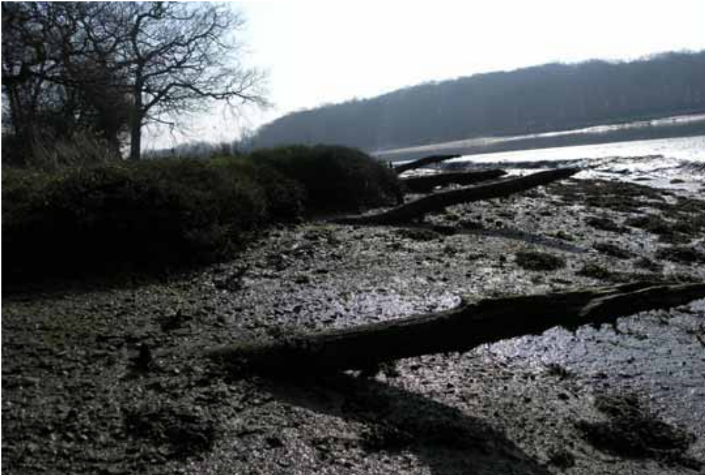
Figure HAM010 - 4 HAM 009 consists of five horizontal timbers protruding from the eastern bank to form part of a wharf or hard
