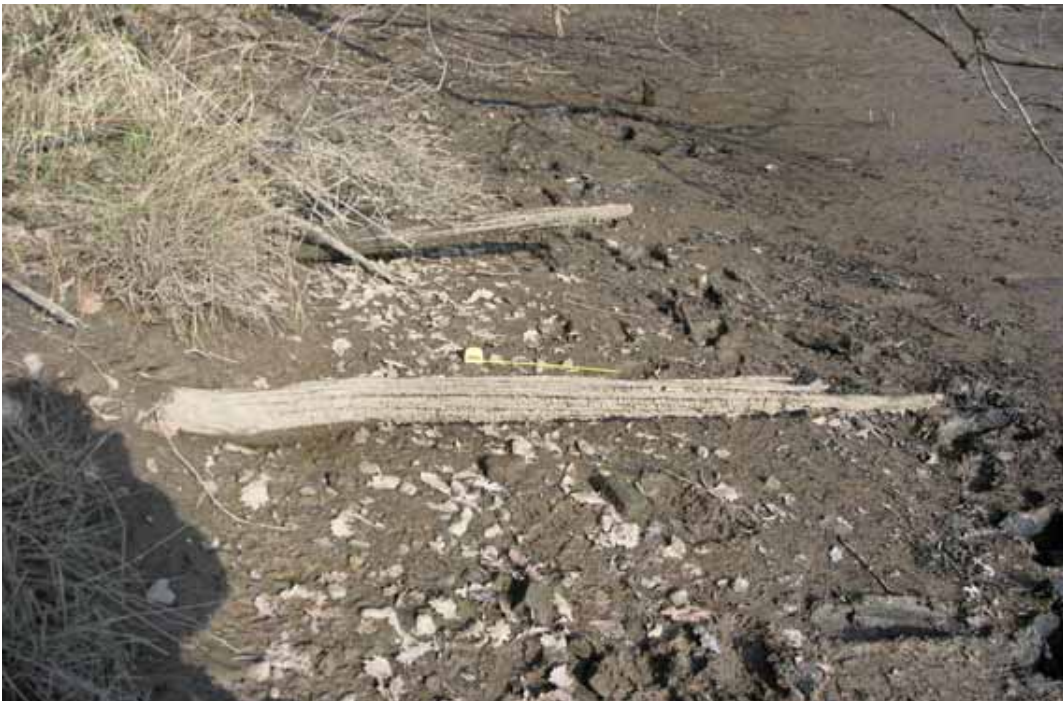
Figure HAM010 - 5 HAM 011 forms the wharf or hard on the western bank where the timbers are more decayed and the revetment less obvious
