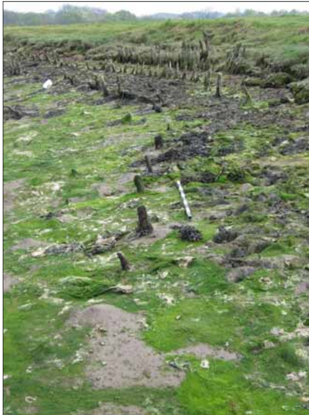
Figure HAM002- 4 Groups 1-9 are located on the southern bank and probably represent a number of structures (Courtesy D. Hopkinson)
