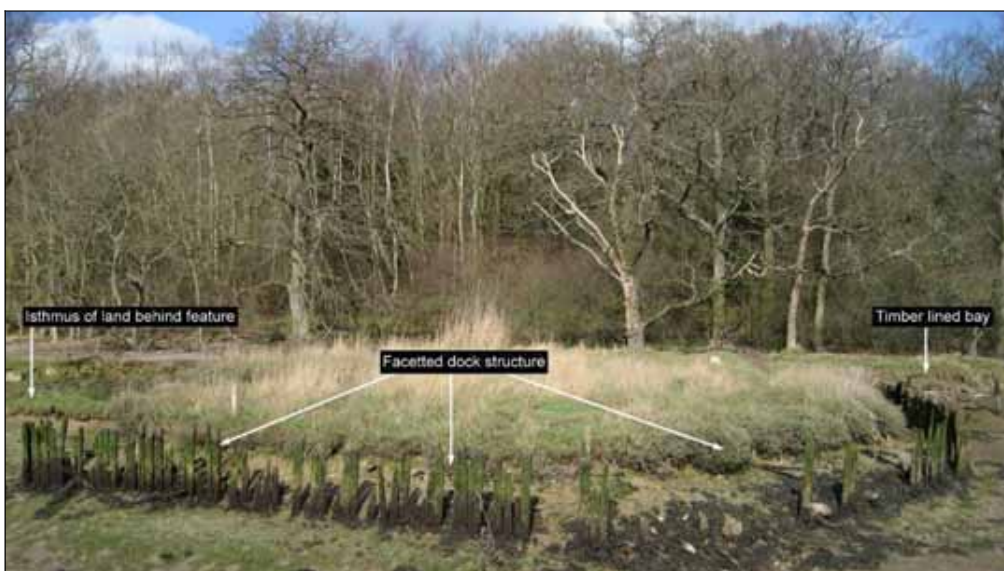
Figure HAM002- 8 The posts form a revetment of varying states of repair surrounding an earth promontory (Courtesy D. Hopkinson)
