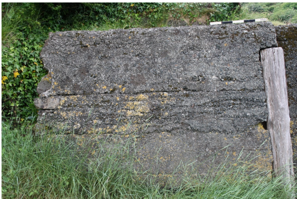
FIGURE 4 - REMAINS OF STONE QUAY
