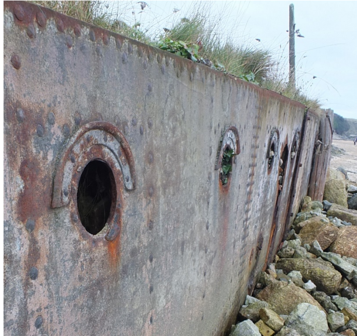
Figure 17: Reinforcements above portholes
