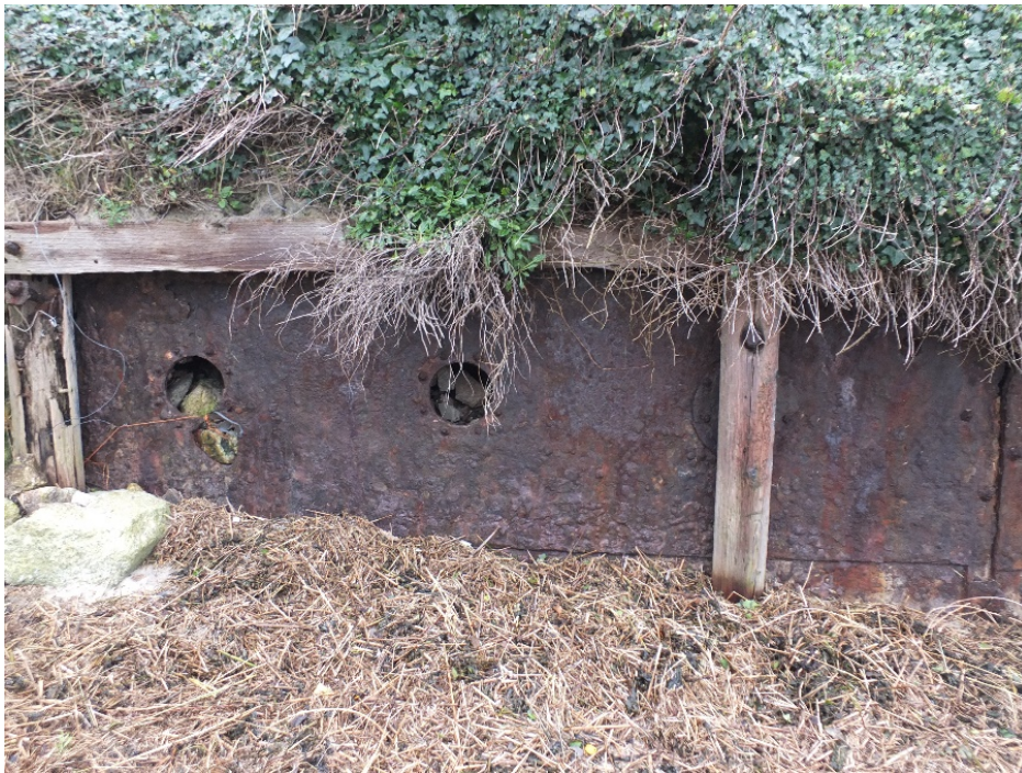
Figure 36: Portholes (one sealed and partially obscured by post) in Section C
