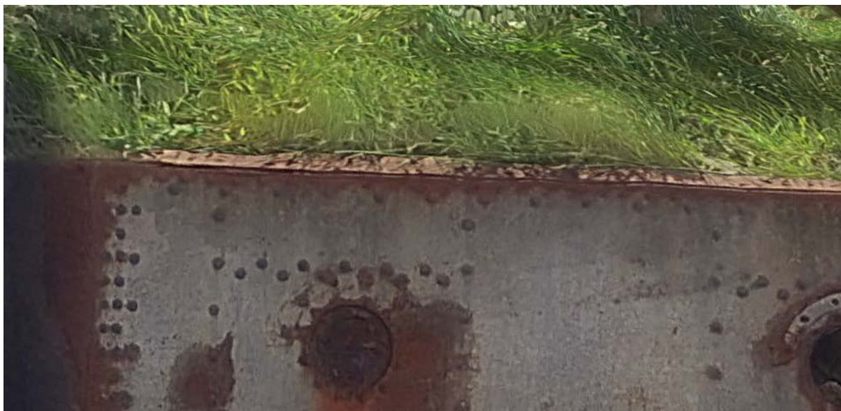
Figure 26: Gunwale riveting pattern Panel 10
