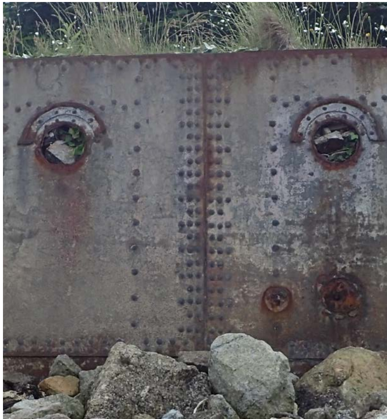
Figure 14: Treble chain riveting pattern for vertical joins
