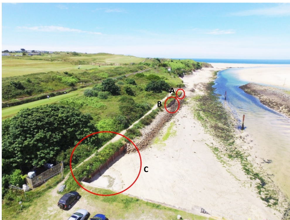
Figure 7: Lelant estuary, sections of ship hull revetment circled, Lelant/Dynamite Quay at bottom of photo (2016)
