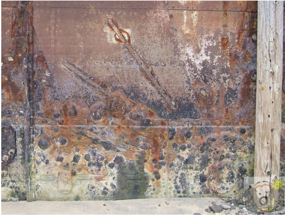
Figure 34: Damage to ship's hull plating (Photo by Raymond Forward 2009)
