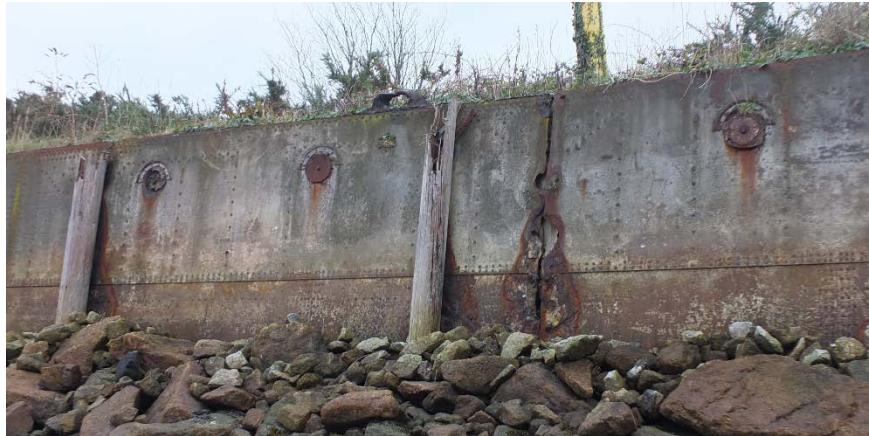
Figure 29: fairlead on gunwale of Panel 14, Section B
