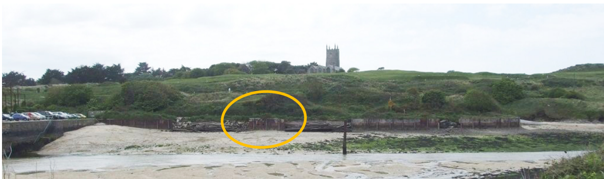
Figure 31: ship hull revetment at Lelant Quay (Photo by Raymond Forward 2009)
