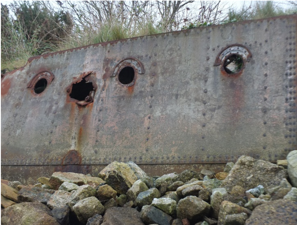
Figure 15: Horizontal joins – double riveted lap joint
