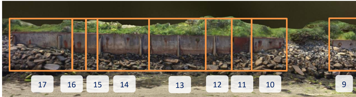
Figure 25: Revetment Section B (Panels 10 - 16)
