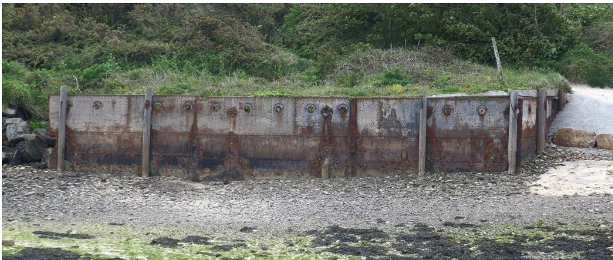
Figure 9: Northern most section of revetment (Photo by Raymond Forward 2009)
